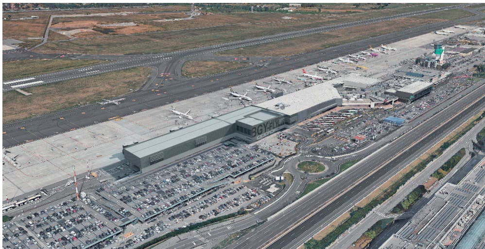
Concept design of expansion of Passengers Terminal of Bergamo Orio al Serio Airport – Italy
