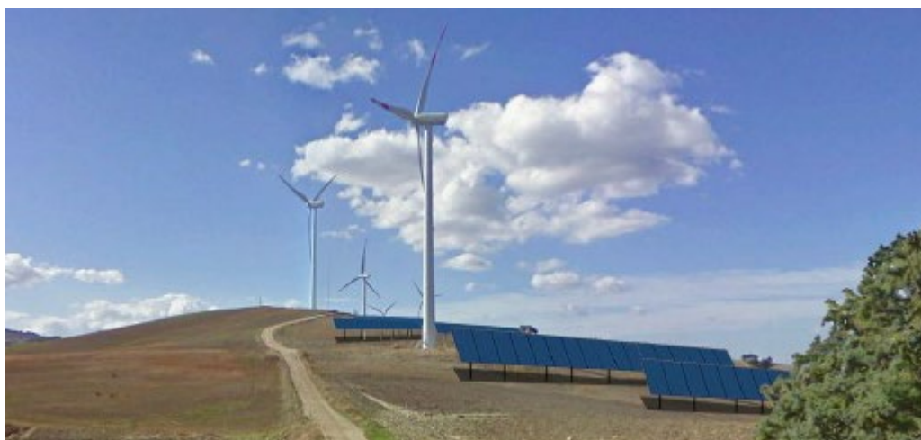
Rotello Solar power plants, Italy
