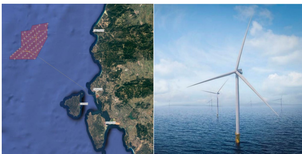
Off shore wind Farm in Sardinia, Italy
