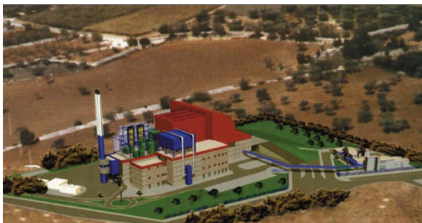
Lecce waste to energy plant
