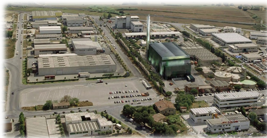
Leghorn waste to energy plant
