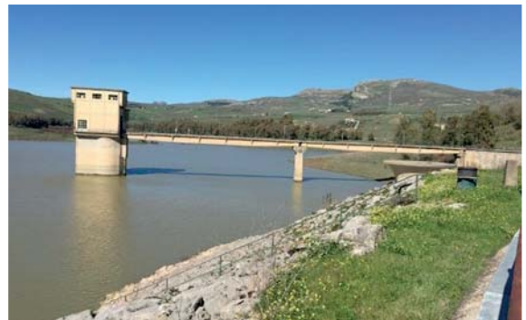
Intake-tower and access bridge
