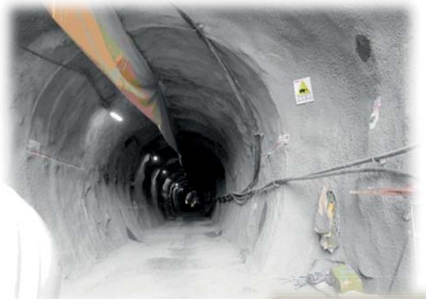
Bottom discharge tunnel
