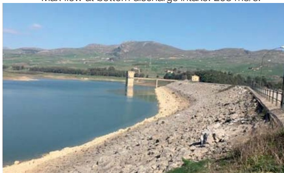
Scanzano dam - general view (inside the bank)
