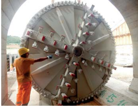
Detail of the TBM
