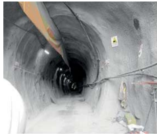
Bottom discharge tunnel of Misicuni Dam
