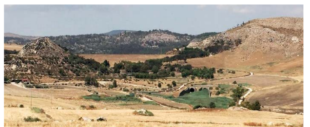
The Disueri Dam (downstream view), in foreground, the two outlet tunnels and the discharge Channel
