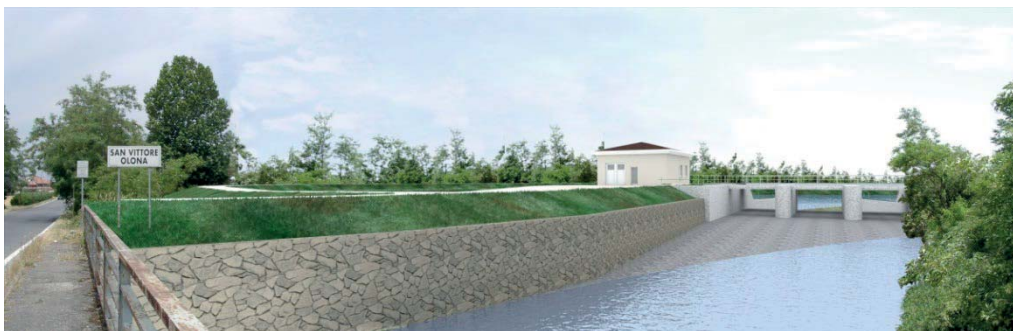
Discharge works on Olona river
