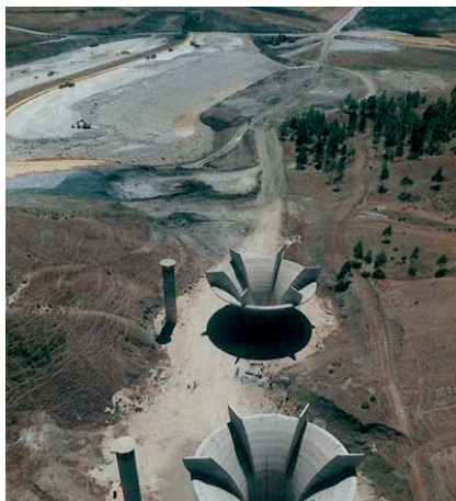
Morning glory spillway Gibbs Dam
