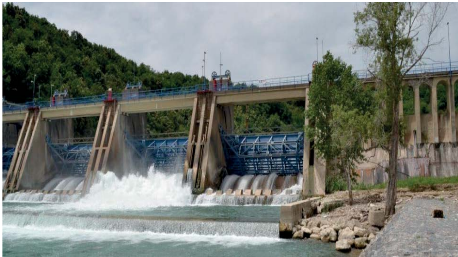
Upgrading of Persano Dam
