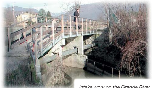
Intake work on the Grande River
