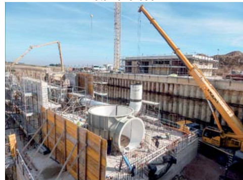
Detail of the main pipe construction
