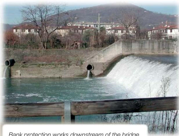
Bank protection works downstream of the bridge
