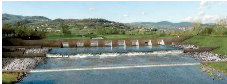
Eight gates connection structure
