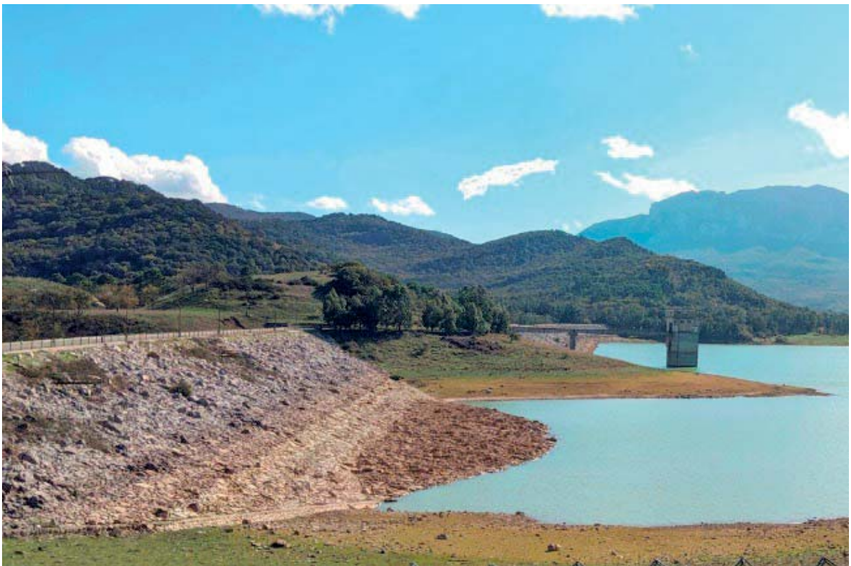
Rossella Dam (inside the bank)
