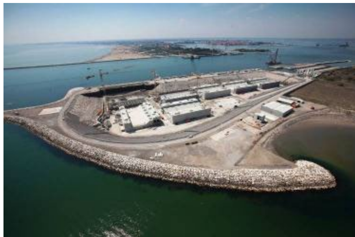
Chioggia inlet – Precast caissons yard
