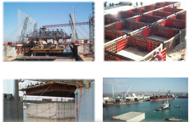
Typical phases of construction, launching and transportation of prefabricated elements
