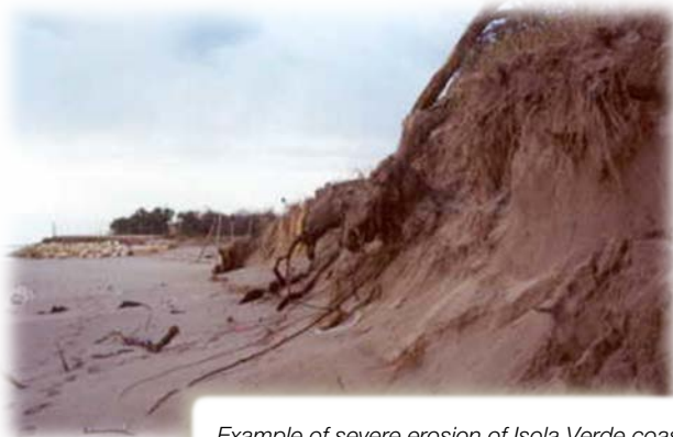
Example of severe erosion of Isola Verde coast
