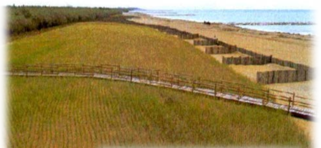
Reconstruction of the coastal dune system
