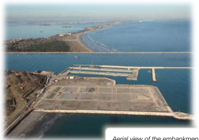
Aerial view of the embankment
