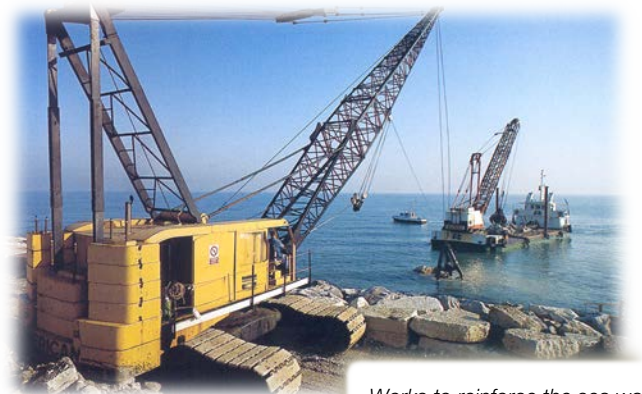
Works to reinforce the sea wall
