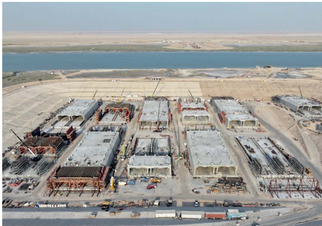
Caissons under construction - Al Faw Port, Iraq
