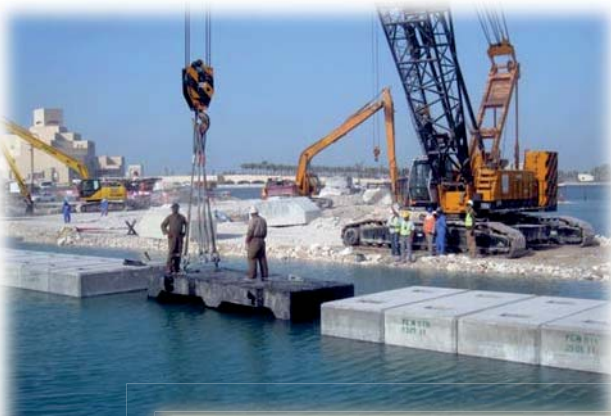
Quay walls construction: laying precast box culvert.
