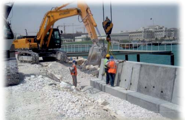
Breakwaters: laying precast crest wall block.
