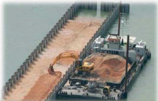
Construction phases of the navigation locks: filling of the cofferdam
