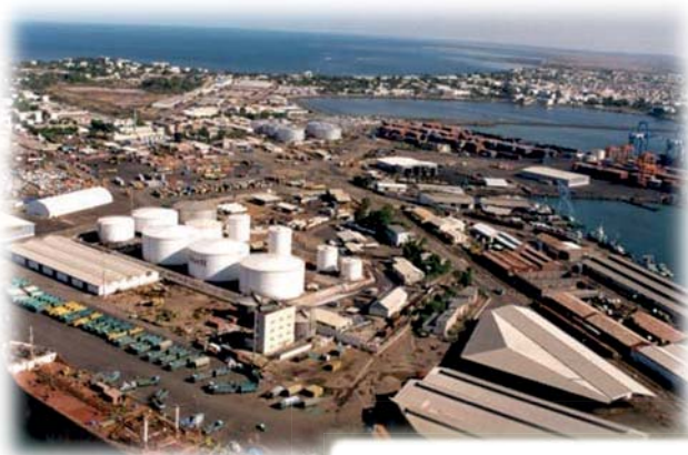
View of the existing oil storage area
