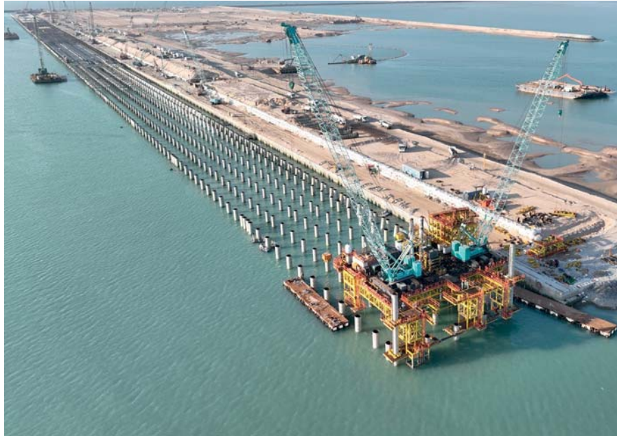
Front view of quay wall - Al Faw Port – Iraq
