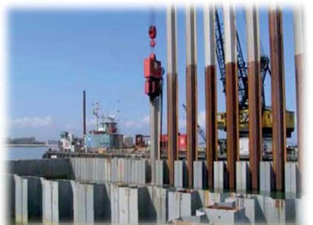
Construction phases of the navigation locks: sheet pile driving
