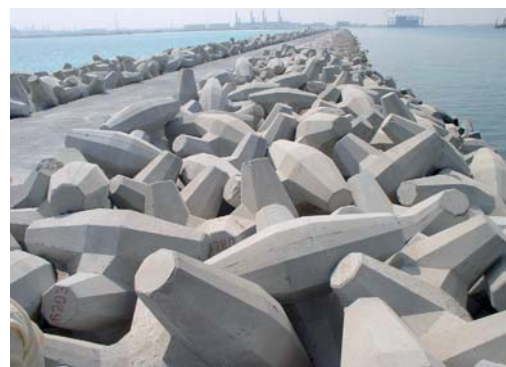
Breakwater – Port of Ras Laffan -Qatar
