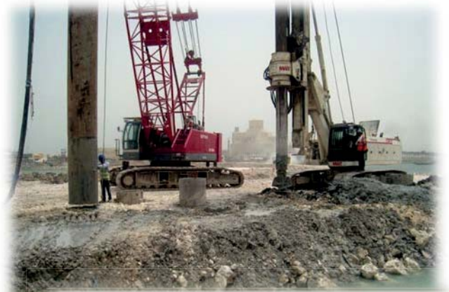
Stone columns soil improvement: driving the casing and drilling.
