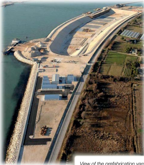
View of the prefabrication yard
