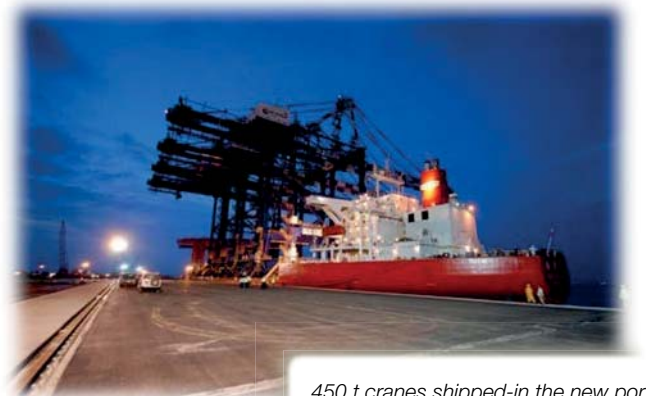
450 t cranes shipped-in the new port
