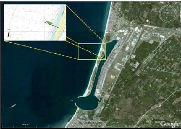
Jetty - Position outside the commercial port
