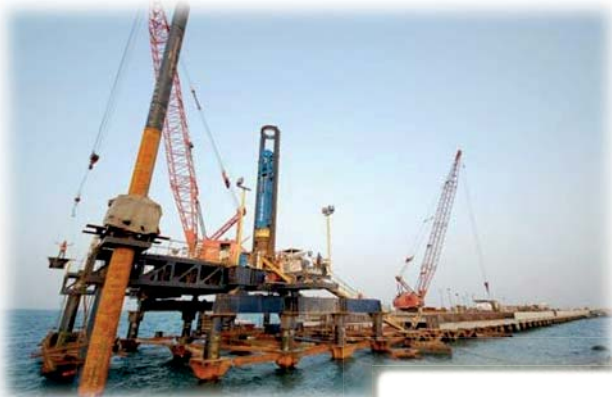
Driving of foundation piles
