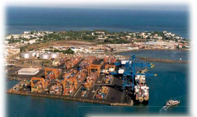
Existing container terminal at Djibouti
