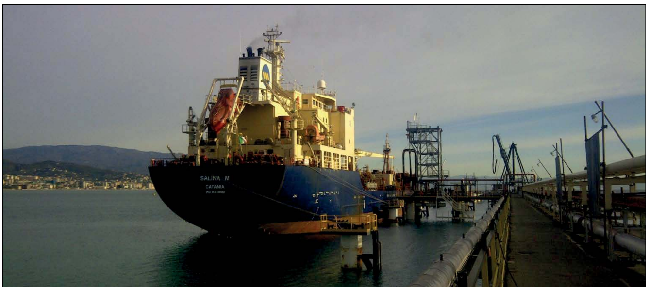
New Exxon berth - View
