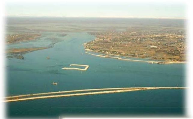
Construction of the central core of Lido island
