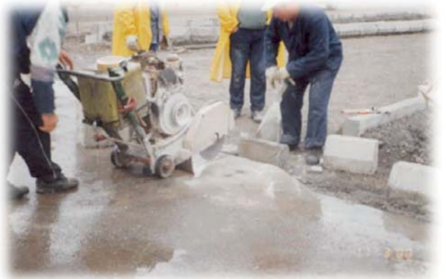
Repair of erosion damages on Railway overpass
