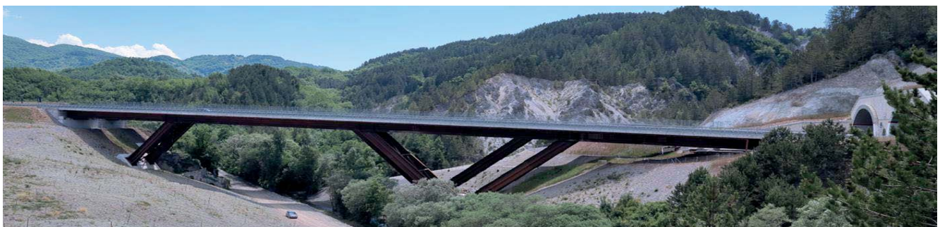
Viaduct Pineta - L= 175 m
