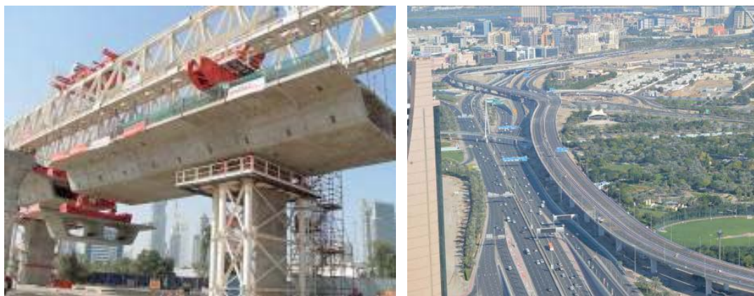
Parallel Roads superstructures – Dubai
