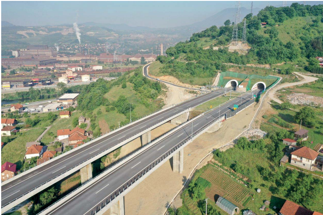
Double carriageways viaducts – Bosnia and Herzegovina
