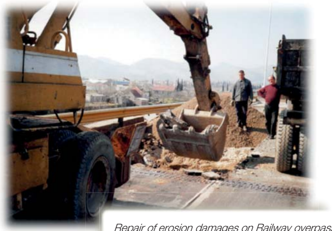
Repair of erosion damages on Railway overpass
