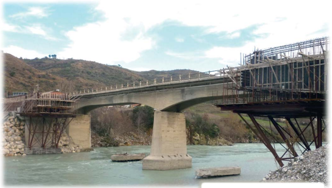
Lot 2 – Bridge under construction at Km 25+185
