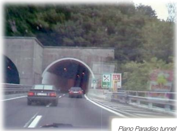
Piano Paradiso tunnel
