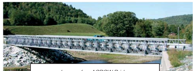
Image of an ACROW Bridge
