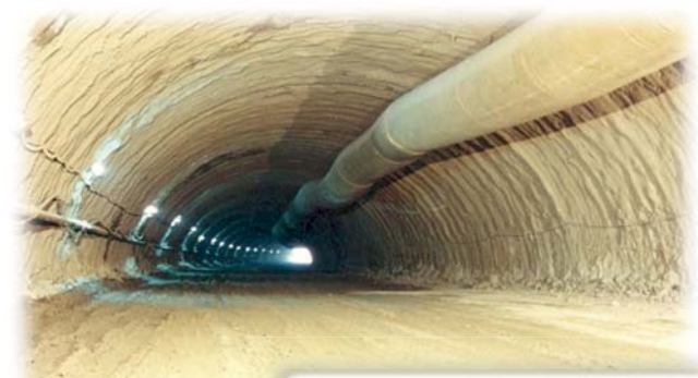
Cozzo Minneria tunnel under construction
