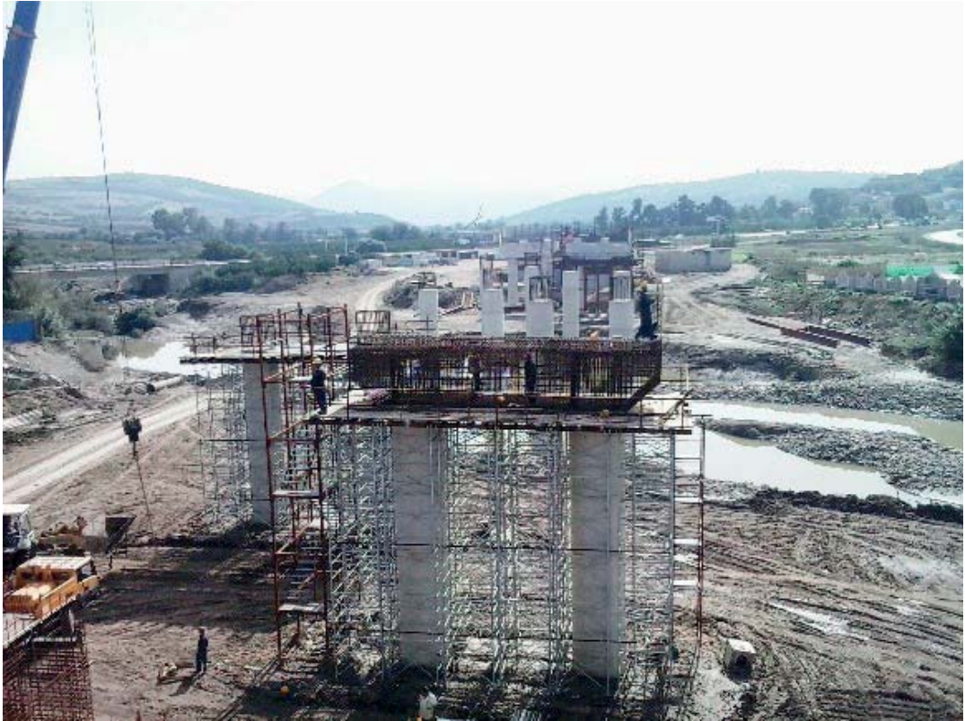
East-West Motorway - Algeria
