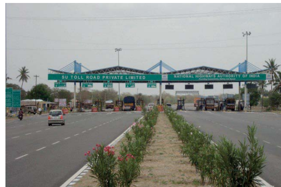
Salem-Ulundurpet motorway - India
