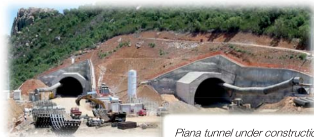
Piana tunnel under construction
