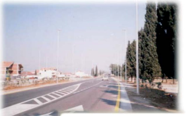
Horizontal signalling and electric lighting completed on the airport road
