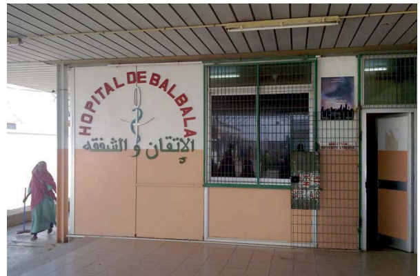
Entrance of the Hospital of Balbala
