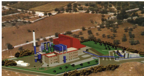
Lecce waste to energy plant
