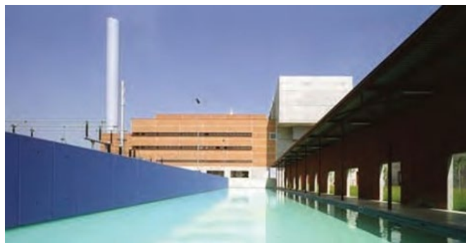
Silla 2 (Milan) waste to energy plant
