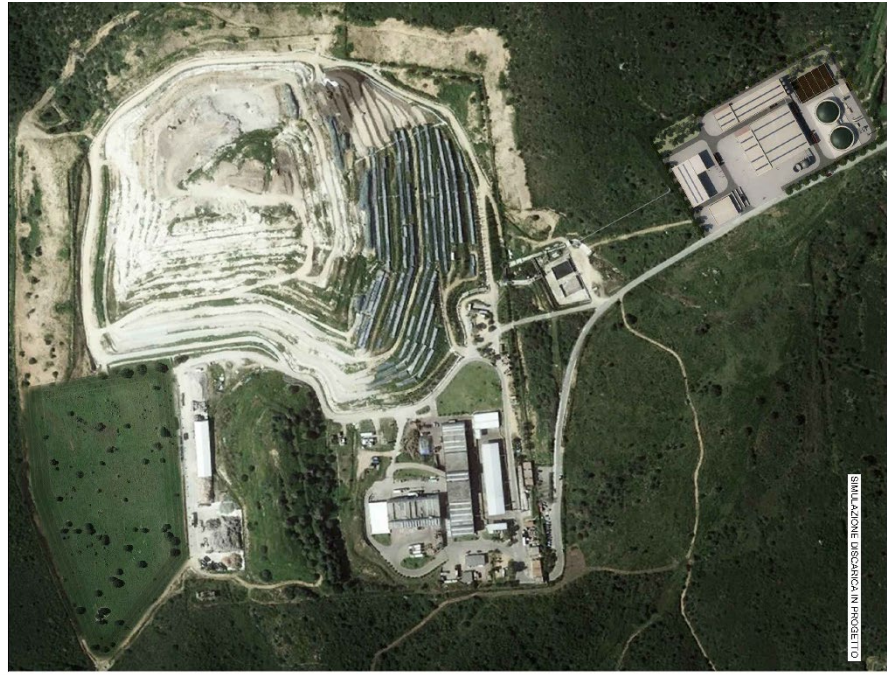
Spirito Santu waste treatment plant, Italy
