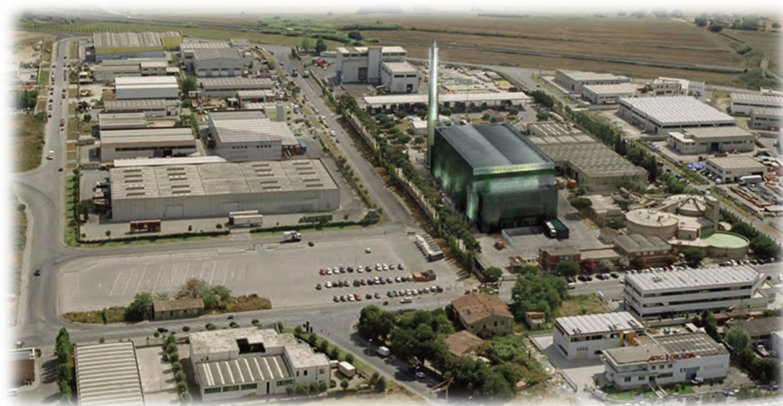
Leghorn waste to energy plant
