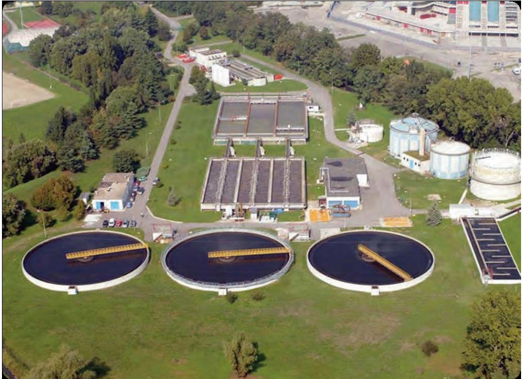
Cesano Boscone, Corsico, Buccinasco and Assago (Milan) wastewater treatment plant
