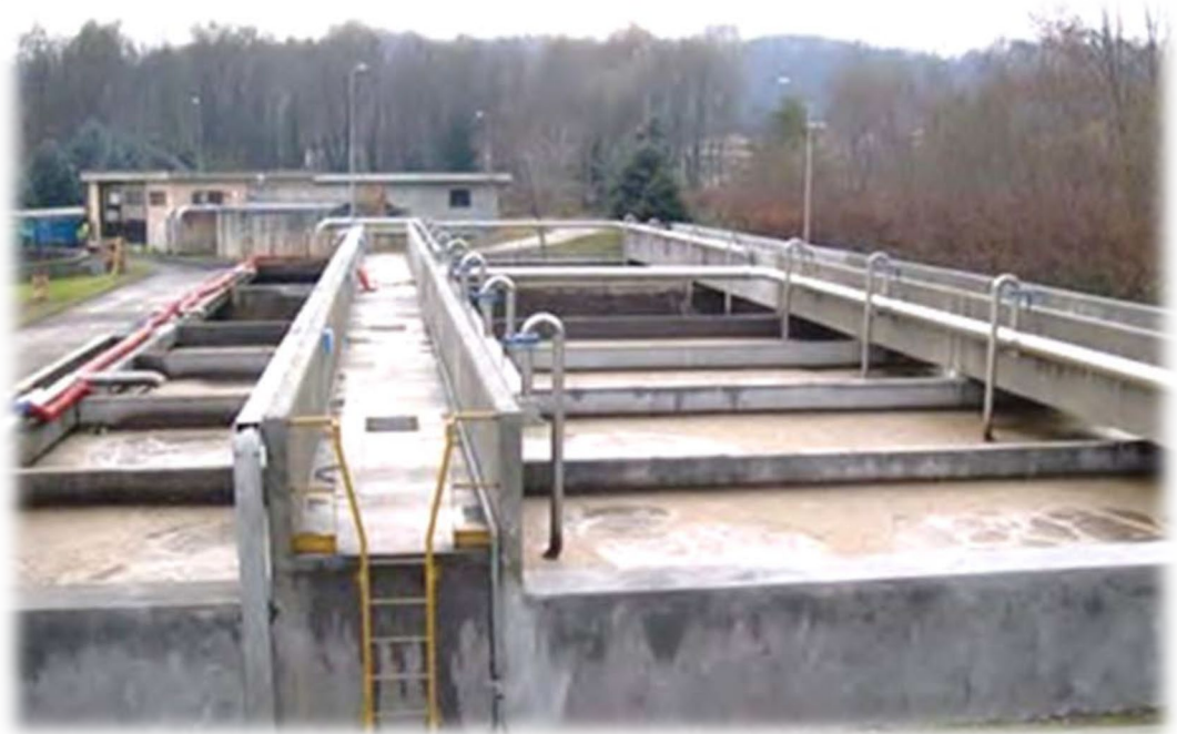
Borgomanero (Novara) wastewater treatment plant
