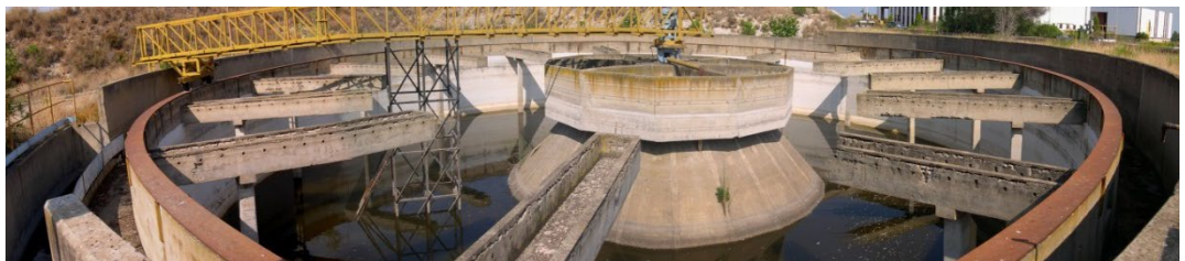
Megara (Syracuse) potabilisation plant
