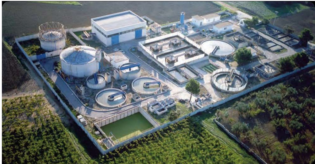
Mottola (Taranto) wastewater treatment plant
