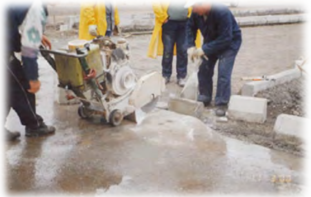
Repair of erosion damages on Railway overpass
