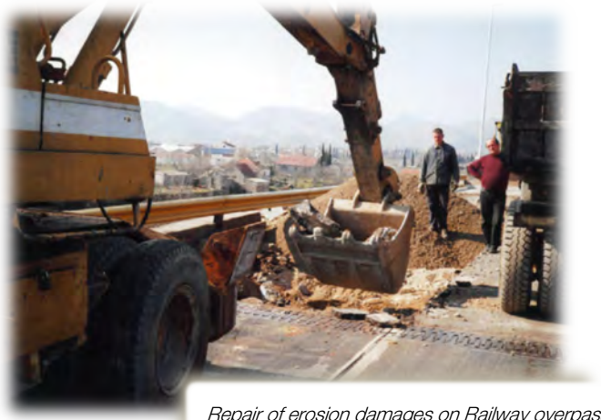
Repair of erosion damages on Railway overpass
