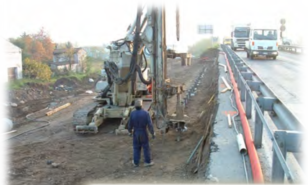
Execution of a sheet-pile for the provisional site works
