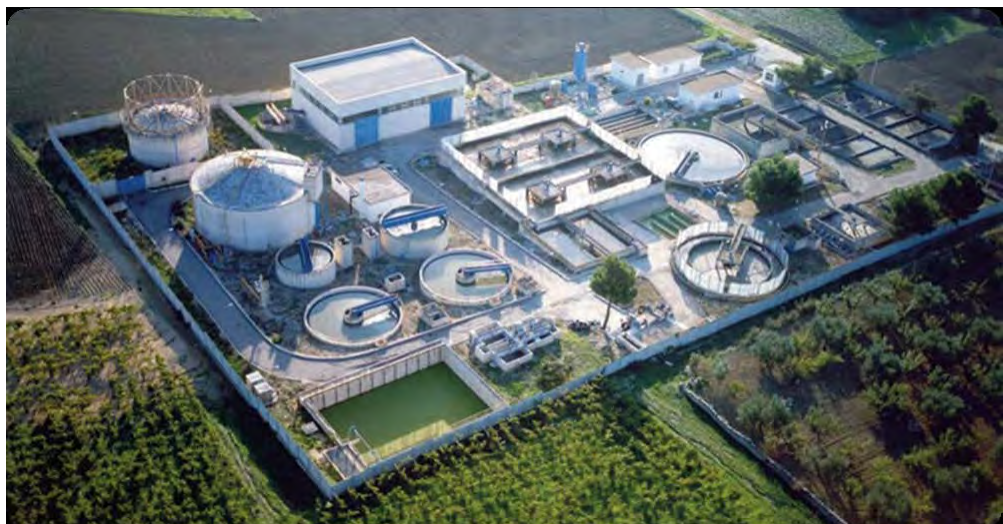
Mottola (Taranto) wastewater treatment plant
