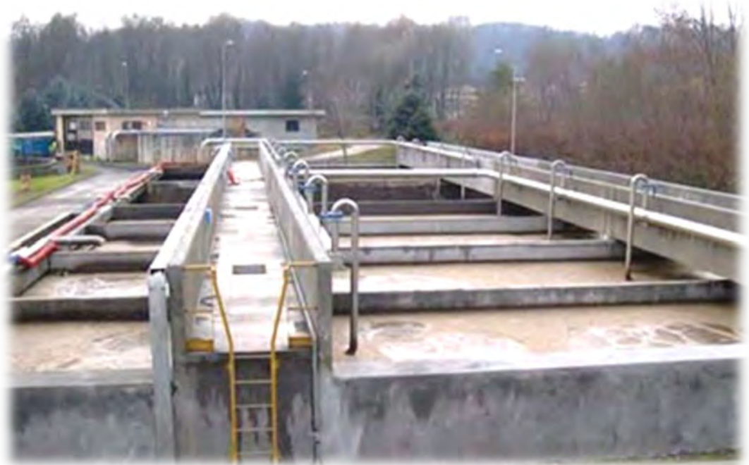
Borgomanero (Novara) wastewater treatment plant
