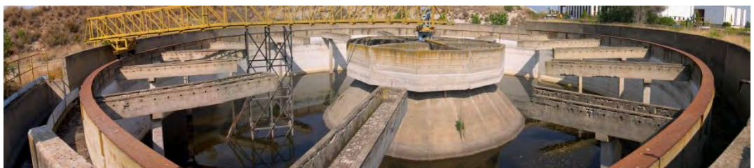
Megara (Syracuse) potabilisation plant
