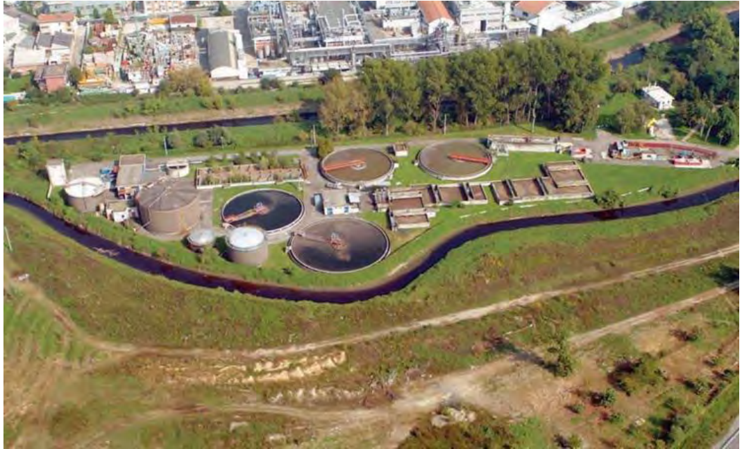
Rozzano (Milan) wastewater treatment plant
